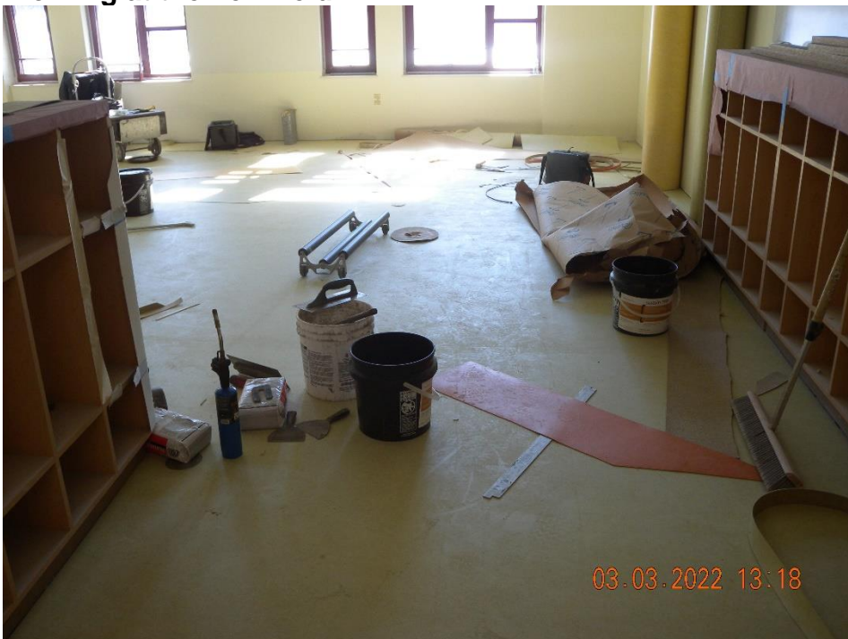
Installing vinyl flooring at building F.
