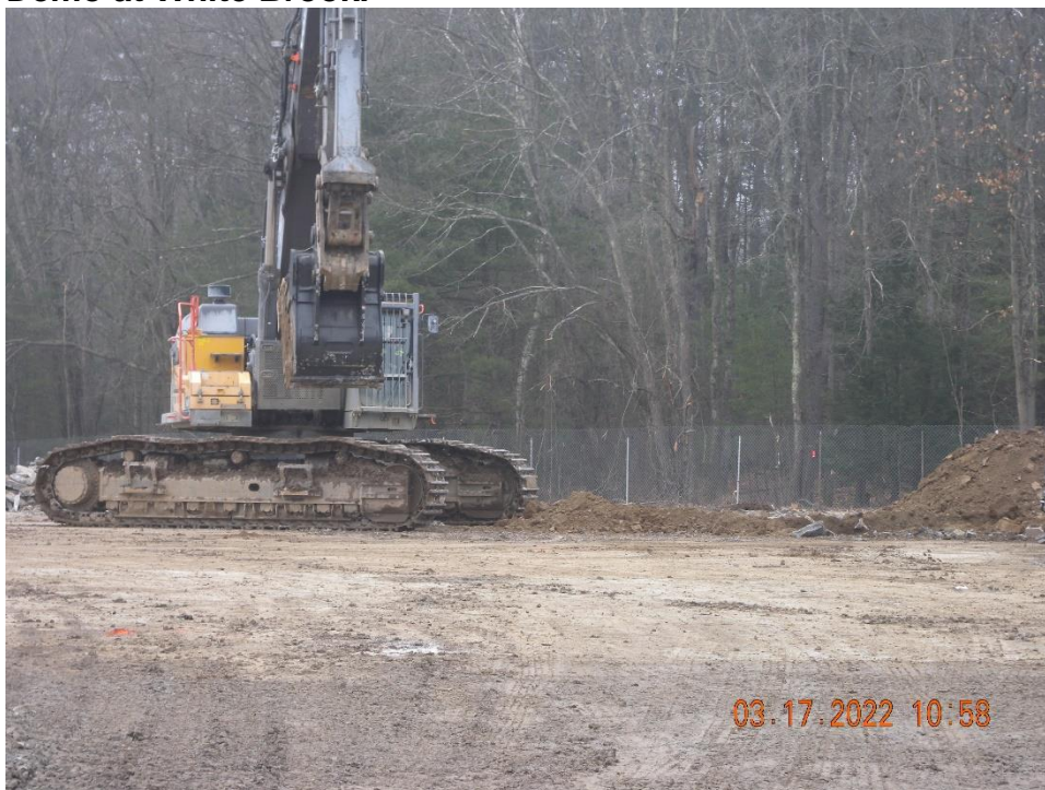
Large excavator removing foundation.
