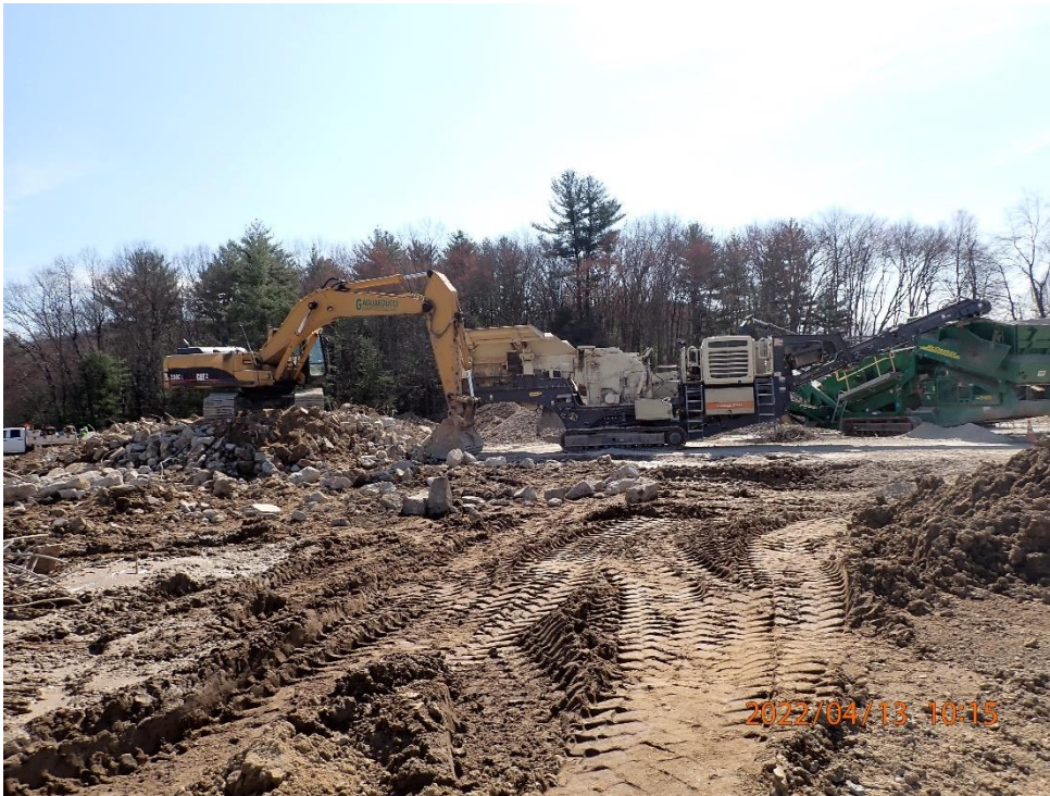
Concrete crushing.
