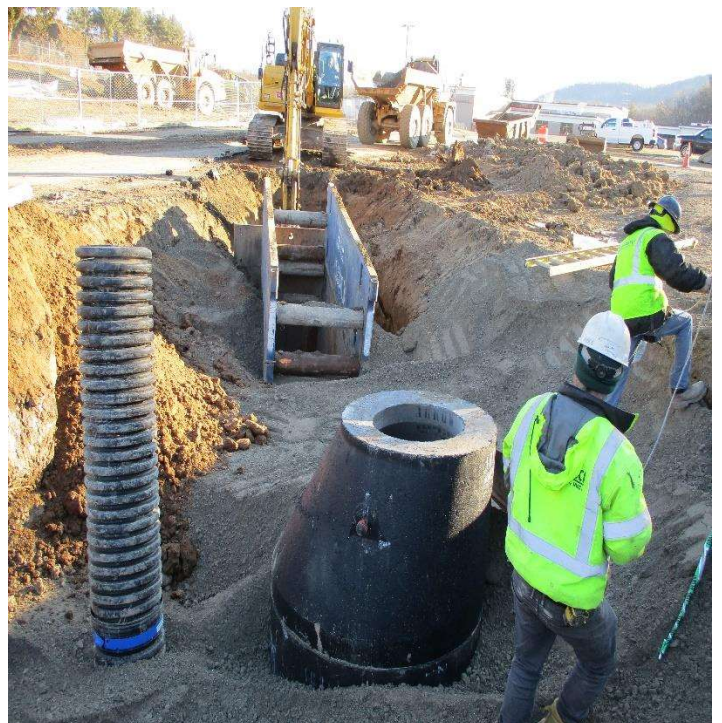
SEWER MANHOLE IN DRIVEWAY ISLAND
