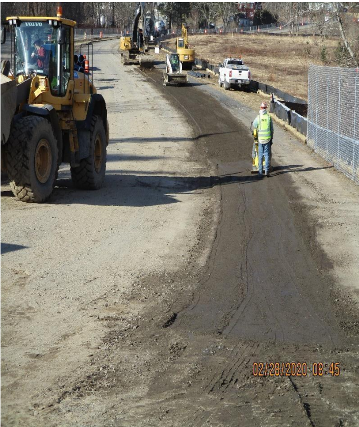
WORK ALONG NORTH SIDE OF NORTH DRIVEWAY
