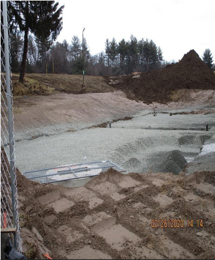
BOTTOM OF RECHARGE BASIN
