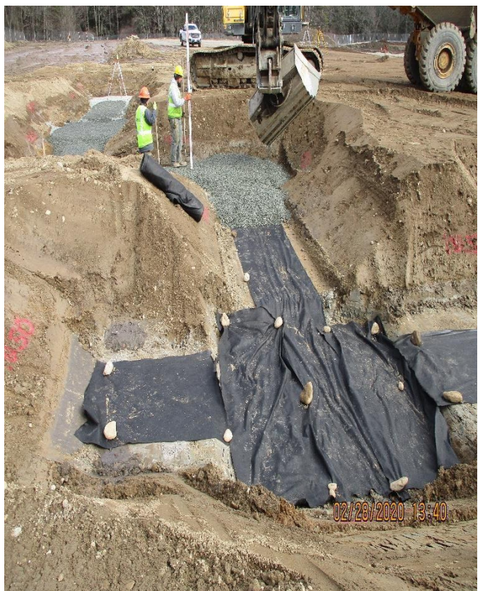
FIRST FOOTINGS EXCAVATED & STONED IN BLDG. C
