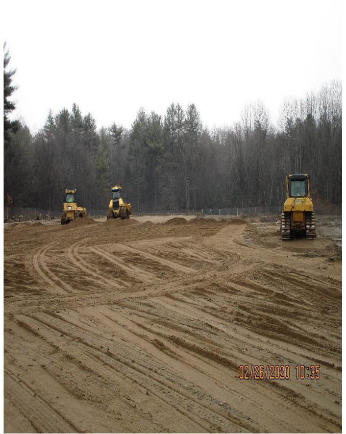
BUILDING-UP THE FIELD GRADE
