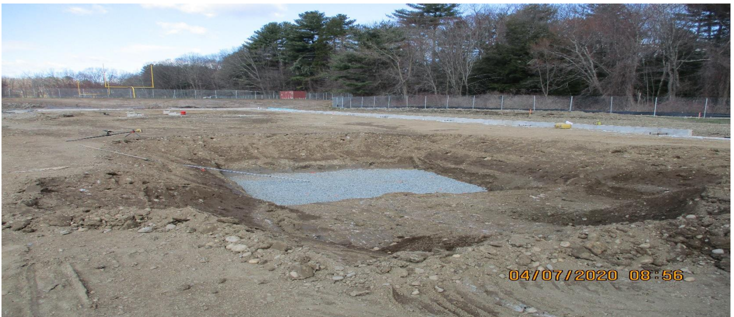
BUILDING B ELEVATOR PIT
