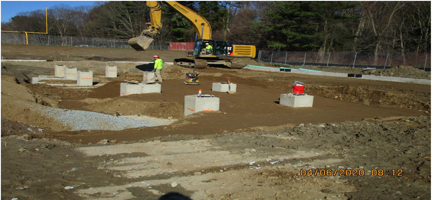
BUILDING B INTERIOR PIERS
