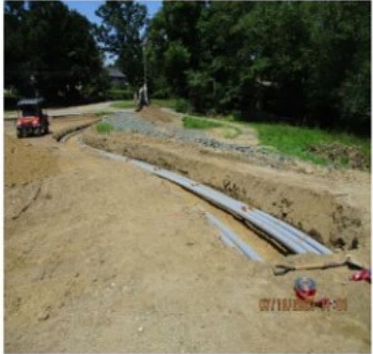
ELECTRICAL DUCT BANK AT ROUNDABOUT (NORTH SIDE)
