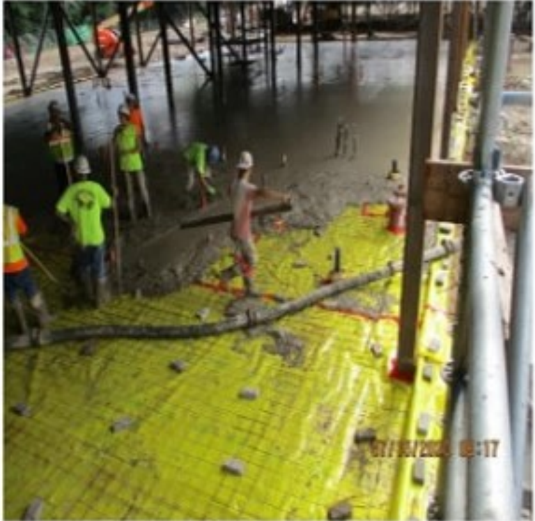
POURING BUILDING B SLAB-ON-GRADE
