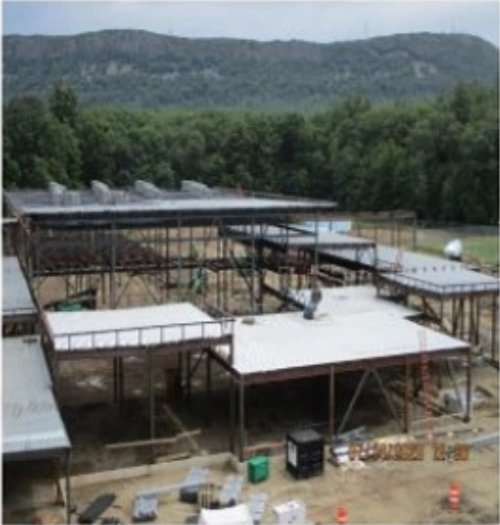
BUILDING A DECKING IN PLACE
